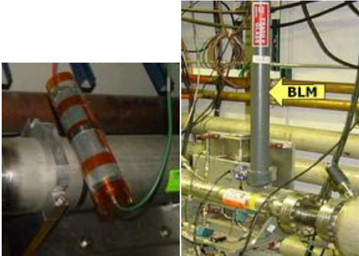
Figure 7.83: Two styles of BLMs will be used. Tevatron-style ion chamber loss monitors (left) will be used in areas of primary beam, and also in the Delivery Ring for Mu2e operations. The Pbar-style ion chamber, which consists of a plastic scintillator and a long light guide connected to a photomultiplier tube shielded from light in PVC, will be used in the Delivery Ring during ( g - 2 ) operations.
