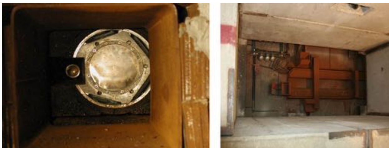
Figure 7.24: (left) Photo of the front face of the beam dump as taken in 2003. (right) Looking down on the top of the dump plug below the surface of the shielding blocks .
