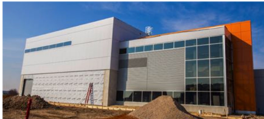
Figure 1.5: The completed MC-1 building in May 2014.
