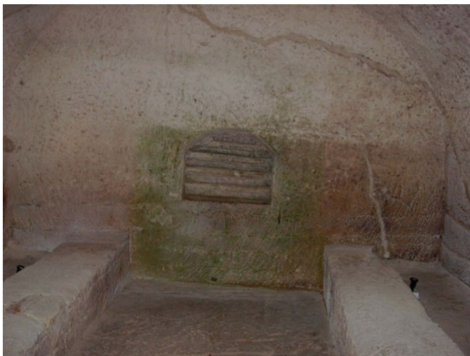
Fig. 6 Reuse of rainwater from Sassi in Matera
