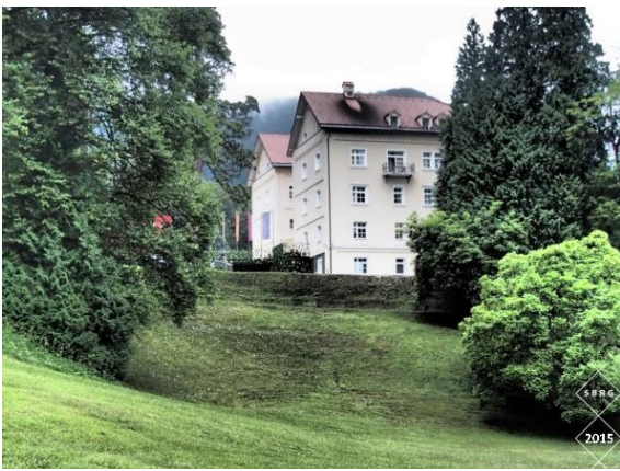
Figure 1. The Rimske Terme Hotel Spa built right on top of the ancient Roman baths and integrates also the original tanks. It is nestled in the wood and has a large garden.
