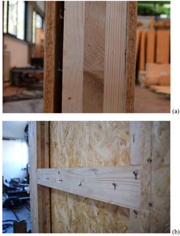
Figure 8: Details of the HTF-2 wall specimen.
