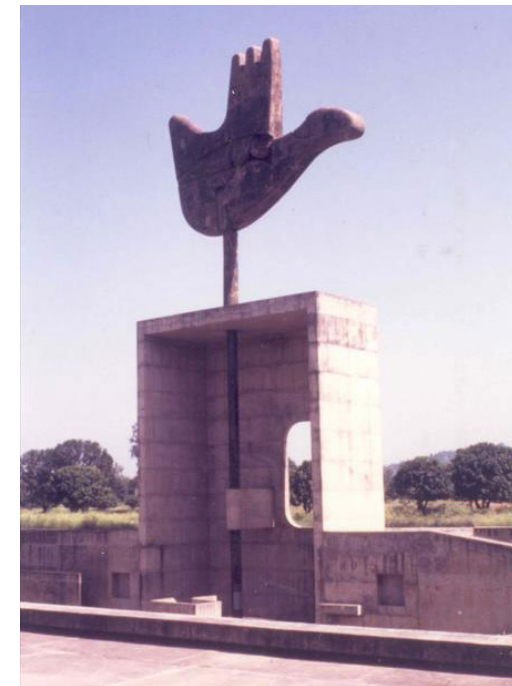
MAIN OUVERTE, CHANDIGARH, INDIA, 1950 - 1965
