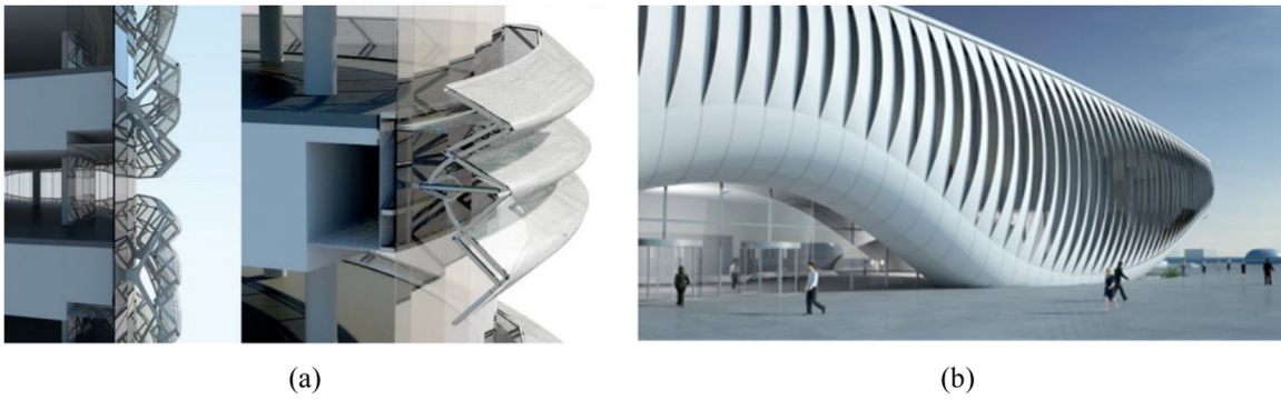
Fig. 1. Examples of constructed adaptive facades: (a) CJ Cheiljedang R&D center, Seoul, South Korea (adapted from [18]) and (b) One Ocean Pavilion, Yeosu, South Korea (adapted from [18]).
