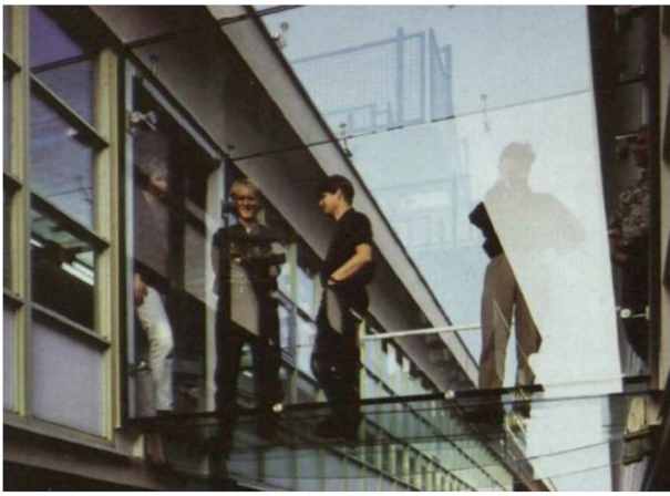
Fig. 1. Example of glass footbridge in Rotterdam (NL, Copyright © HG Esch).
