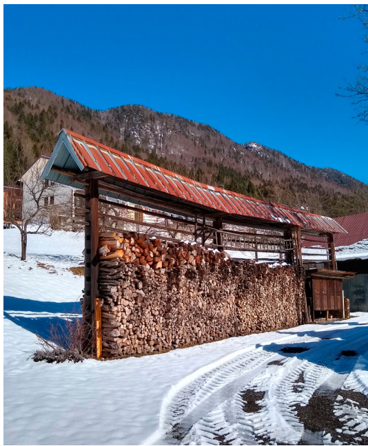
Figure 11. 'Köse', an agricultural construction for drying hay; now repurposed as a shelter for firewood (own photo, 2020).
