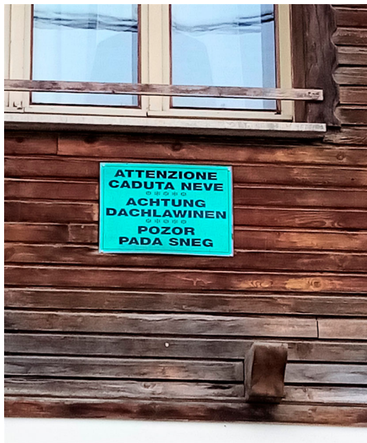
Figure 8. Multilingual sign warning of roof avalanches (own photo, 2020).
