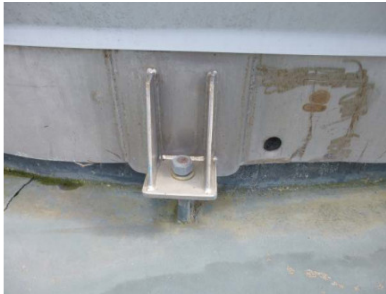
Figure 1.2: Example of plinth-mounted steel tank anchorage [3].
