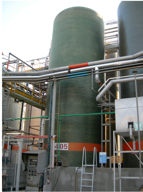
Figure 1.1: Slender fiberglass tank ( H/R = 6 ), filled with 100\text{ m}^3 of Hydrochloric Acid 33% solution.
