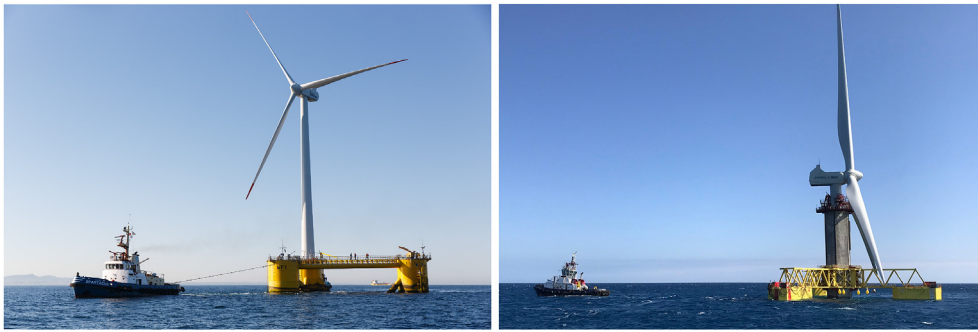
Fig. 1. Towing maneuver of WindFloat unit, left (credits to Recharge, Oslo, Norway) and ESTEYCO's ELICAN, right (credits to ESTEYCO).
