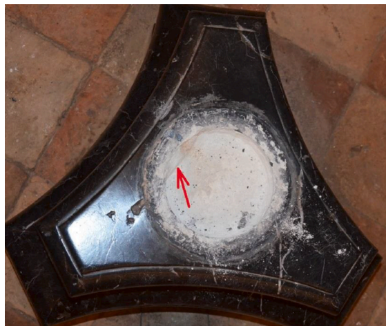
Fig. 4. Stone prominence of the basement mortise.
