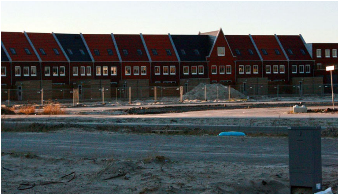
Figure 4. The new town of Almere under construction. (Photo: Yannis Tzaninis)
