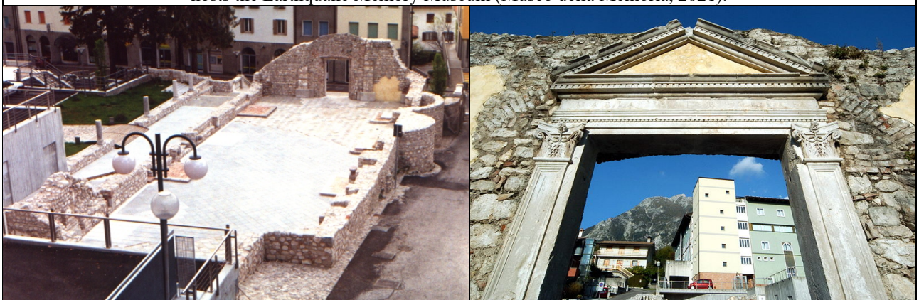
Figure 2b. The restored ruins of the Madonna delle Grazie Church (plant: left; portal, right), completely destroyed by the 1976 Friuli earthquake (Cragnolini, 2012).
