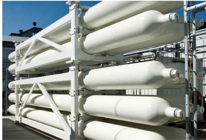
Figure 162. Large diameter seamless steel cylinders. [125]
