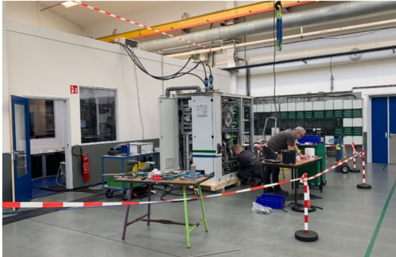
Figure 76. Overview of system test setup. [110]
