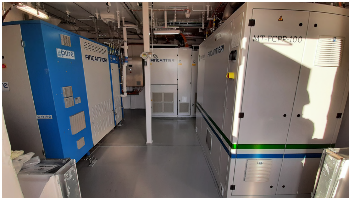
Figure 176. Onboard demonstrator. Fuel cell rom. Photo by the author.
