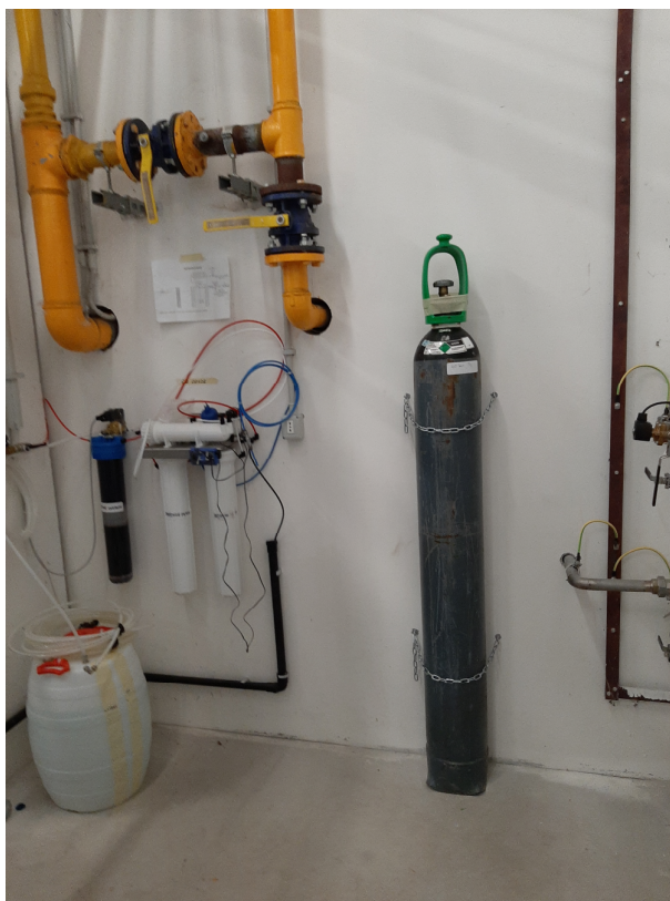
Figure 142. Electrolyser demineralized water tenk (left) and nitrogen cylinder (right). Photo by the author.
