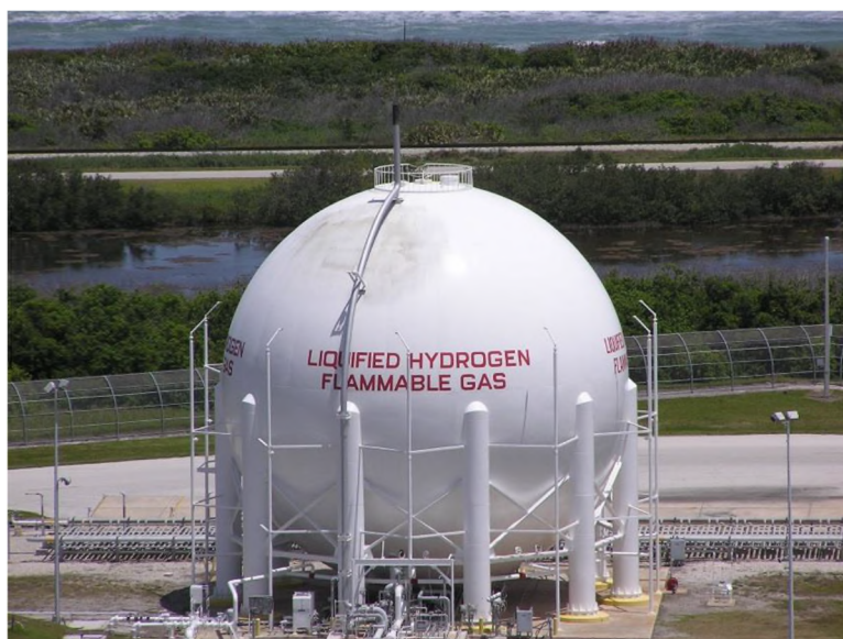
Figure 48. Kennedy Space Center hydrogen tank. [79]
