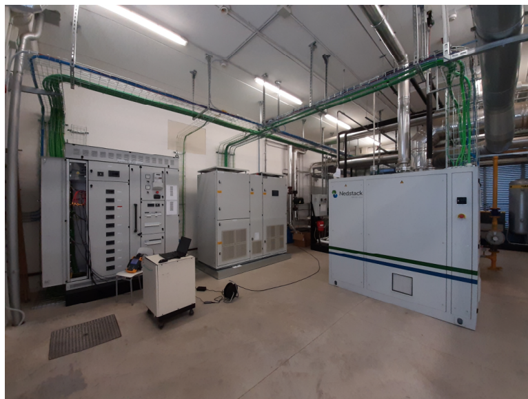
Figure 144. Fuel cell generator during electrical power plant characterization tests. Photo by the author.
