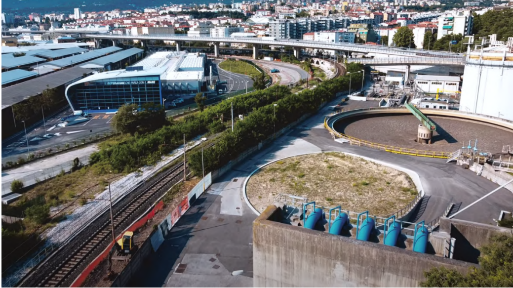
Figure 24. The WWTP of Servola (Trieste, Italy)
