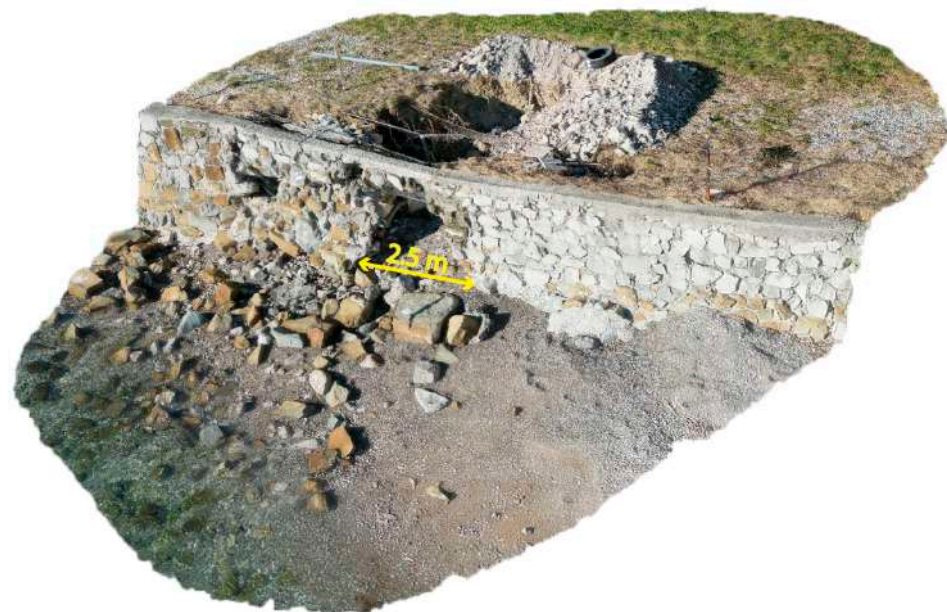
Figure 11. Three-dimension model of the sinkhole H on 29 November 2023 ( https://skfb.ly/p7Uzu , accessed on 21 August 2024). It was already partially filled with landfill material. The retaining wall is almost completely broken. View towards the north-west. The ground resolution of the model (provided by the Agisoft Metashape report) is equal to 3.34 mm/pix.
