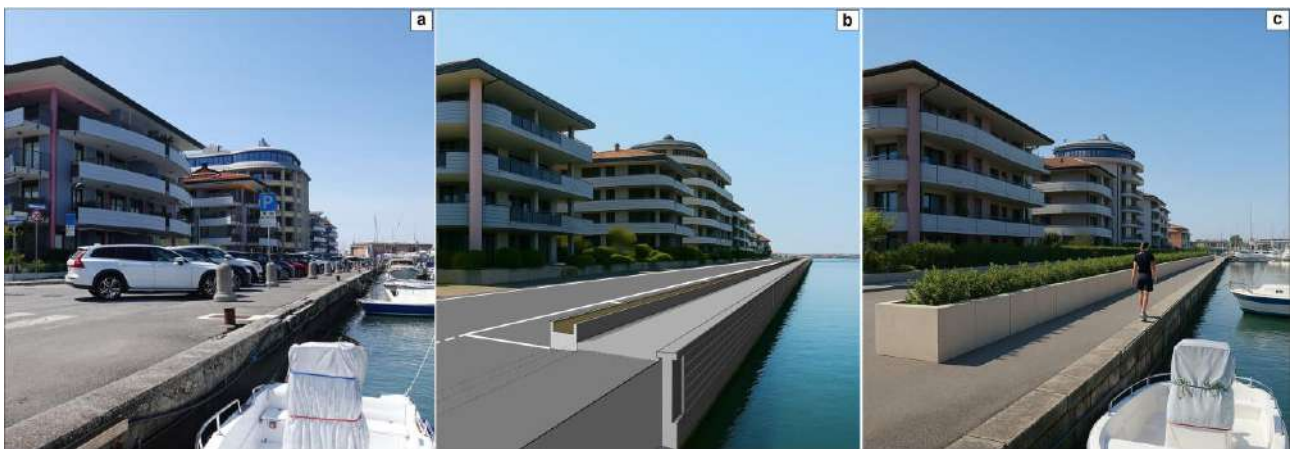
Figure 61. The Riva Brioni promenade. (a) Photo of a promenade section, taken at coordinates 45°68'28.63" N, 13°38'06.56" E (photo credits: Spadotto S.). (b) Design of a bulkhead planter system, built along the entire promenade. Toward the lagoon, the promenade is maintained. Toward the street, parking spaces are created parallel to the bulkhead planter, and the roadway is maintained. (c) Rendering of what Riva Brioni might look like. For the sake of clarity, possible regulated openings needed between the planters for pedestrian transit and dock access are not depicted here.
