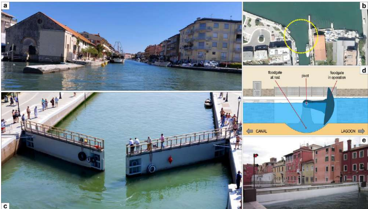
Figure 62. The Mandracchio Canal docks. (a) View of the Mandracchio C. lagoon entrance (Photo credits: Fontolan G.). (b) Plan view of the Canal opening. (c) Example of Porte Vinciane (Da Vinci's gates) mobile system for flood defence in Cesenatico, a Project by Binini Partners ( www.bininipartners.it ). (d) Functional design of Baby Mo.SE floodgates in Chioggia (after ( www.bininipartners.it ) modified). (e) Example of mobile floodgate in operation in Chioggia (after (Il Baby MOSE, 2015) modified).
