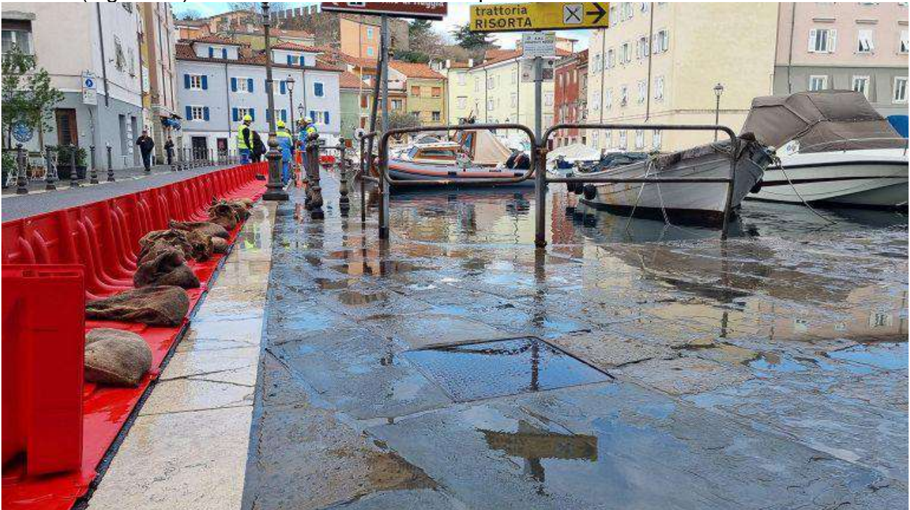
Figure 64. Example of a movable gate barrier applied to the Mandracchio Canal waterfront (Figure 34) (from https://www.rainews.it/tgr/fvg/articoli/2025/01/allerta-meteo-acqua-alta-nel-mandracchio-a-muggia-posizionate-le-barriere-mobili-9f41a40f-4d3b-49c4-8962-29ac1471c016.html ).
