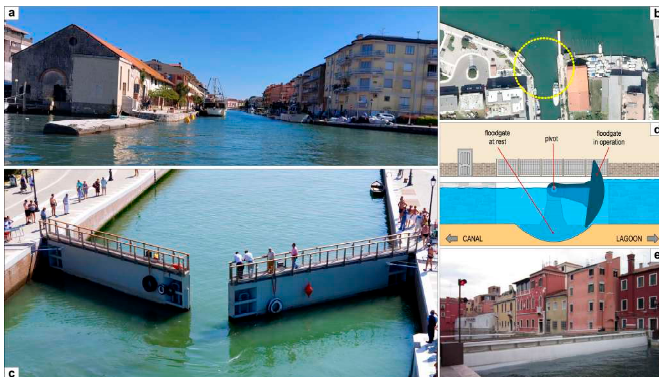
Figure 12. The Mandracchio Canal docks. (a) View of the Mandracchio C. lagoon entrance (Photo credits: Fontolan G.). (b) Plan view of the Canal opening. (c) Example of Porte Vinciane (Da Vinci’s gates) mobile system for flood defence in Cesenatico, a Project by Binini Partners (after [116]). (d) Functional design of Baby Mo.SE floodgates in Chioggia (after [117], modified). (e) Example of mobile floodgate in operation in Chioggia (after [117]).
