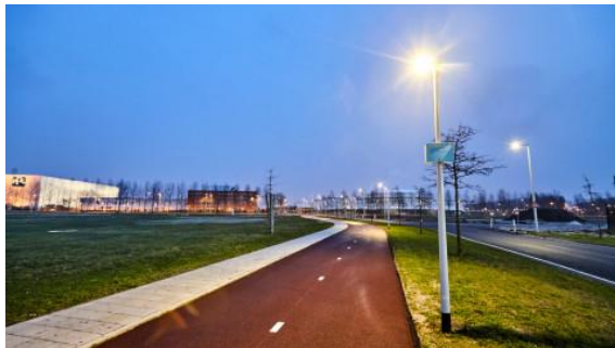
Fig. 2. DC powered lighting system in the port of Amsterdam
