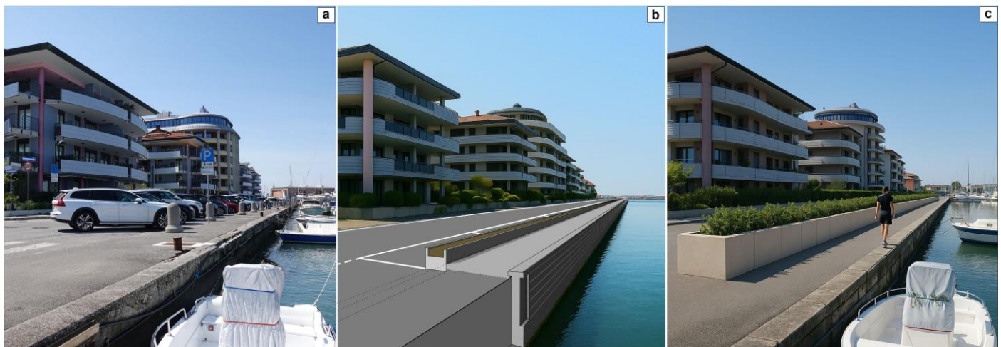
Figure 11. The Riva Brioni promenade. (a) Photo of a promenade section, taken at coordinates 45°68'28.63" N, 13°38'06.56" E (photo credits: Spadotto S.). (b) Design of a bulkhead planter system, built along the entire promenade. Toward the lagoon, the promenade is maintained. Toward the street, parking spaces are created parallel to the bulkhead planter, and the roadway is maintained. (c) Rendering of what Riva Brioni might look like. For the sake of clarity, possible regulated openings needed between the planters for pedestrian transit and dock access are not depicted here.
