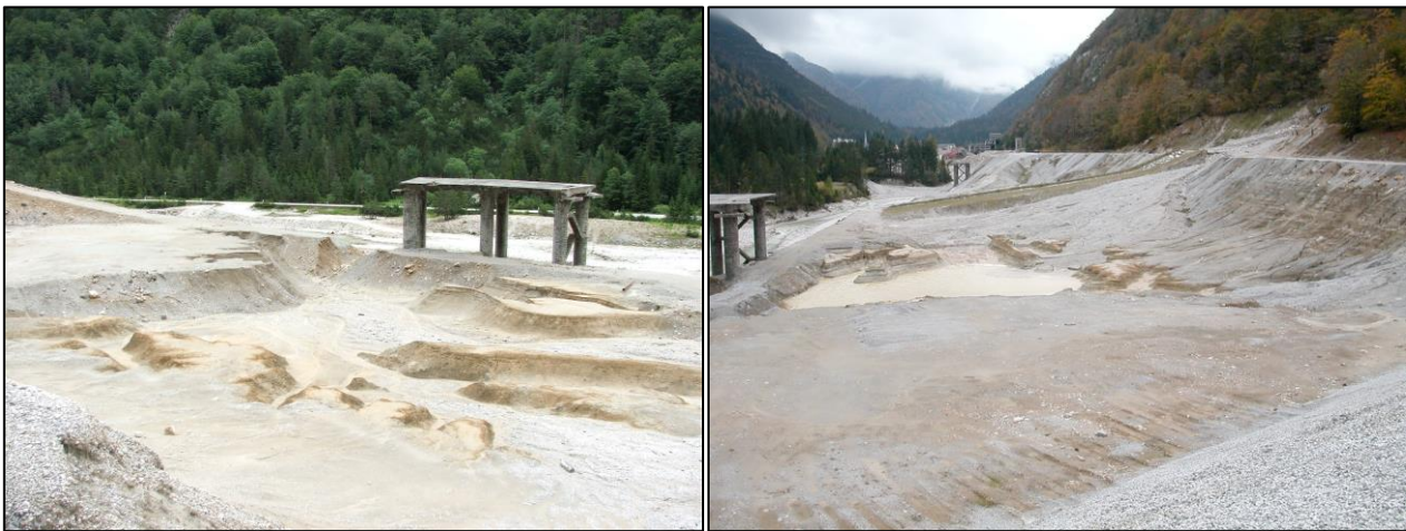
Figure 14 - Tailings pond n° 1. Left: particular erosion of the pond and failure of the dam, right: view from the north (Iadarola and Viso, 2009).
