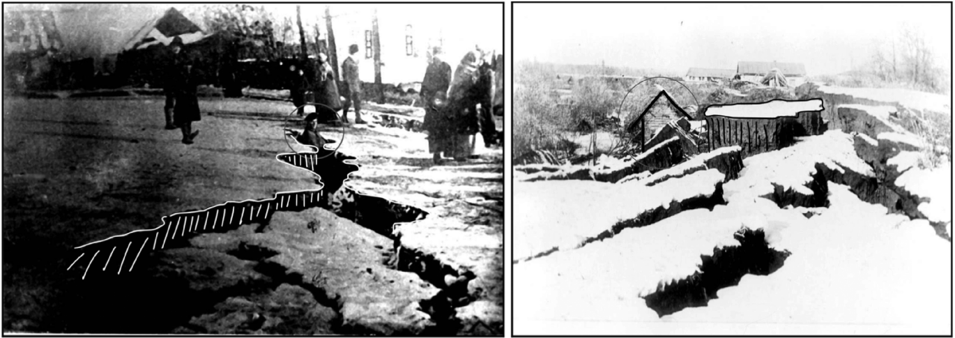
Figure 2. Ground failure effects documented after the 3 January 1911 Kemin earthquake (modified from Nurmagambetov et al., 1999 ).
