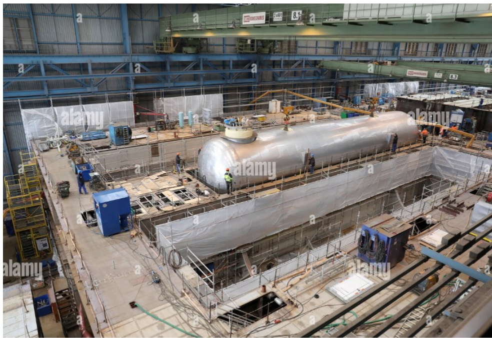
Figure 77 - LNG storage system installation onboard Costa Smeralda [218]
