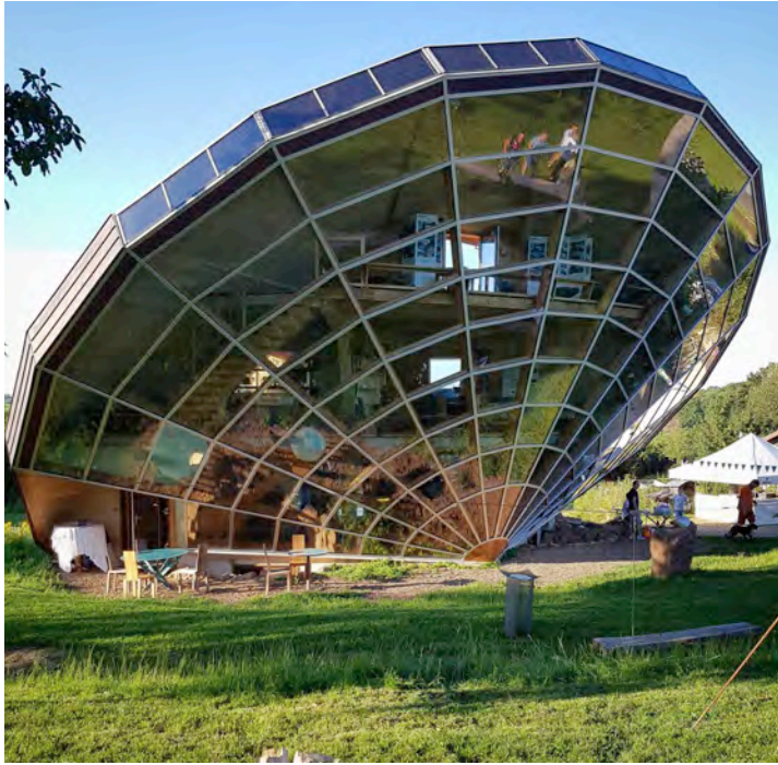
Figure 15. Heliodome is a passive house, one of the most efficient in the world, which exploits the sun's radiant maximisation thanks to its meridian shape, and which follows the sun's trajectory. Eric Wasser, 2013, Cosswiller, France.
