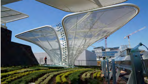
Figures 9-10. Solar textiles applied to tensile structures for Expo 2015 in Milan.
