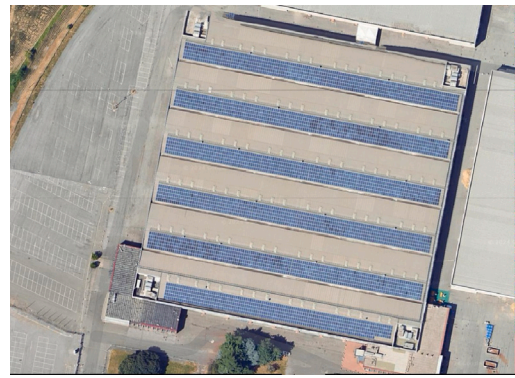
Fig. 1. The PV system under investigation from which the EL images from the PV modules were captured.
