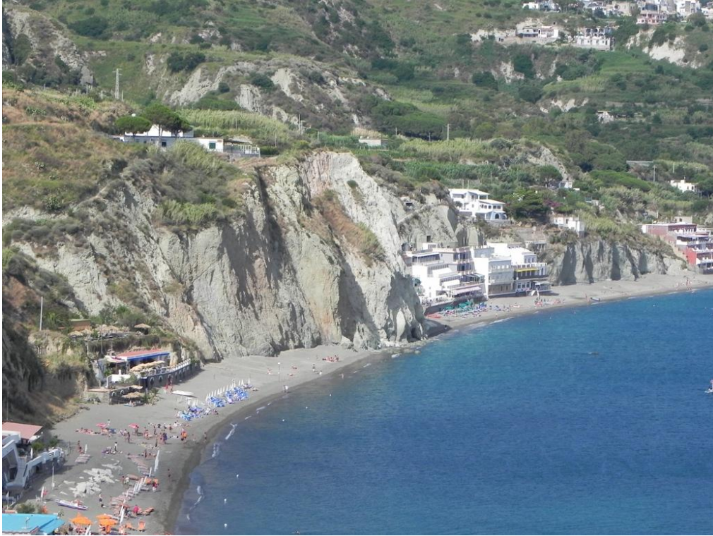
Fig 11. Landslide in Maronti Beach, Barano (Ischia). Source: Eleonora Guadagno, 2024.
