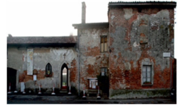
4. Linterno Farmhouse Chapel
