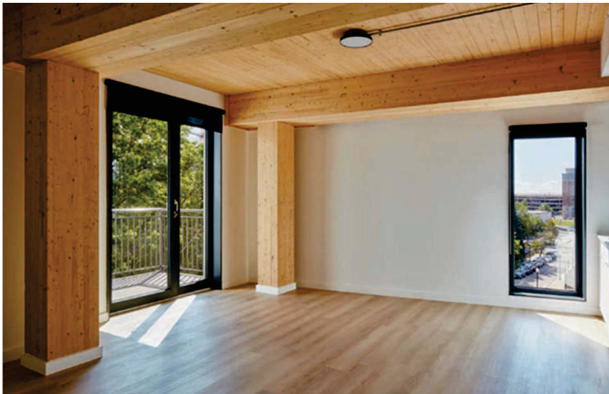
Fig. 7 – CLT flooring (from [20]).
