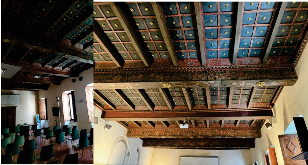
Fig. 115 – Tested timber floor of the historical Palace.
