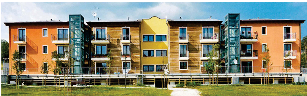
Fig. 6 – Example of CLT building from the CASE project of L'Aquila (image from [4]).
