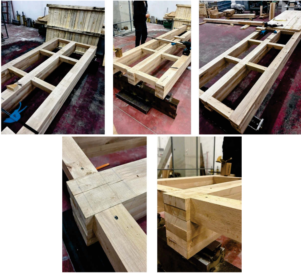
Fig. 45 – Assembling phases of the full-scale timber floor (up) and particular of the secondary joists (down).
