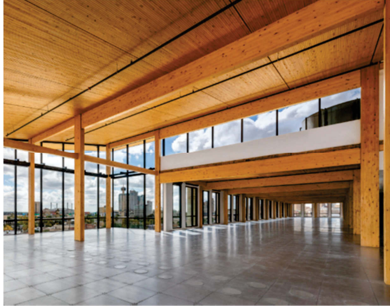
Fig. 8 – GLT flooring (from [20]).
