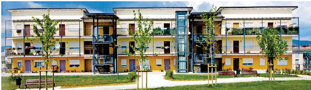
Fig. 2 – Example of Light-Frame Timber building from the CASE project of L’Aquila (image from [4]).
