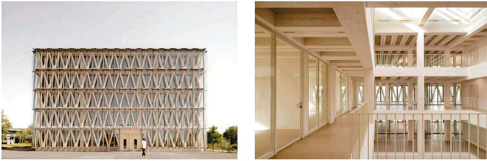
Fig. 4 – Innovation Factory, Hellbronn (Germany), from Waechter Architects.
