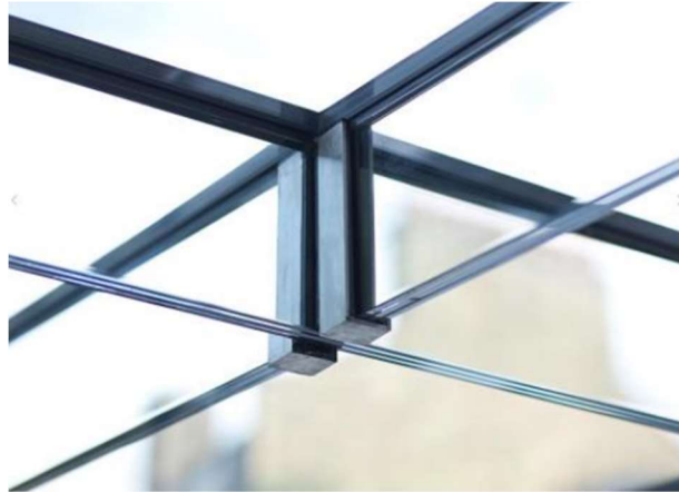
Figure A.1-3 Connection detail between glass beams 1
