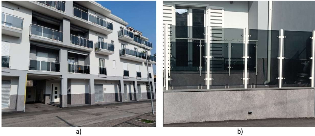
Figure A.1-6 Two practical example of glass balustrades in residential buildings, (photos © S. Mattei)
