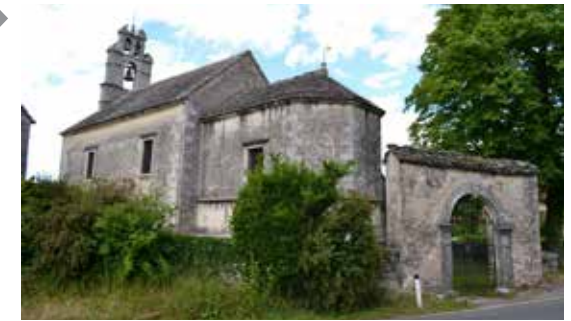
Figure 5.2.7: Church of Our Lady of the Assumption in Šmarje pri Sežani (Photo: Fabiana Pieri)
