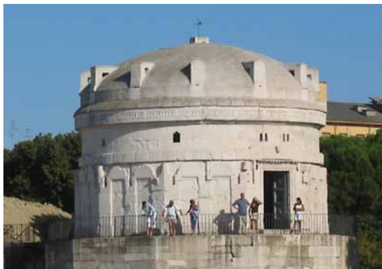
Figure 5.1.4: Mausoleum of Theodoric in Ravenna with a roof, made of a single block of Aurisina-Nabrežina limestone (Photo: Franco Cucchi)
