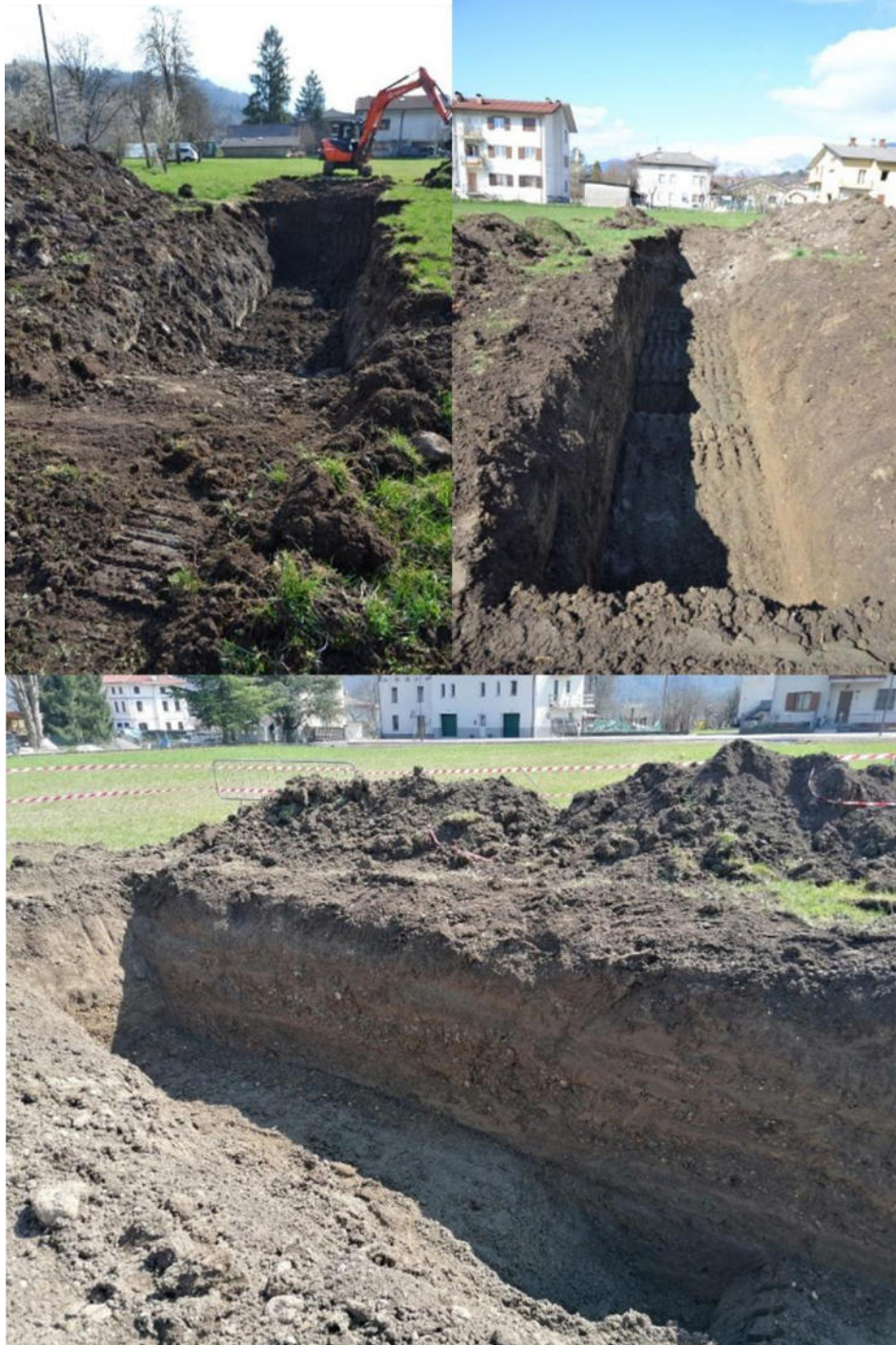
Figure 61 The phases of the trench excavation
