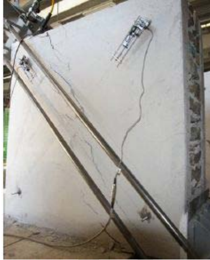
Fig.11. Cracking of the reinforce coating in specimen DC2.
