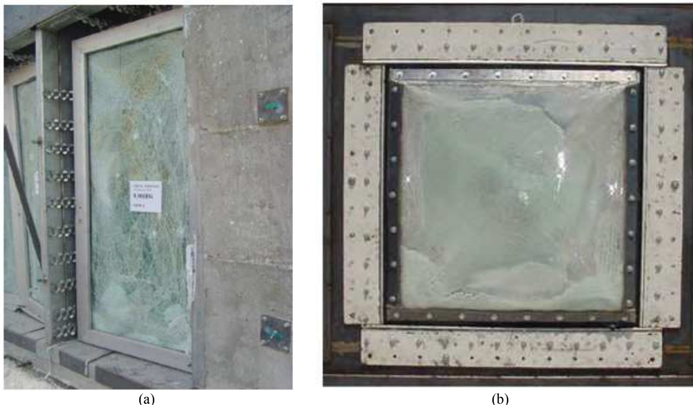
Fig. 12. Blast mitigation with new window frame system. (a) Punched windows with 'sliding boundary' (Zhang and Hao, 2015) and (b) damping chamber system (Trawinski et al. , 2004)
