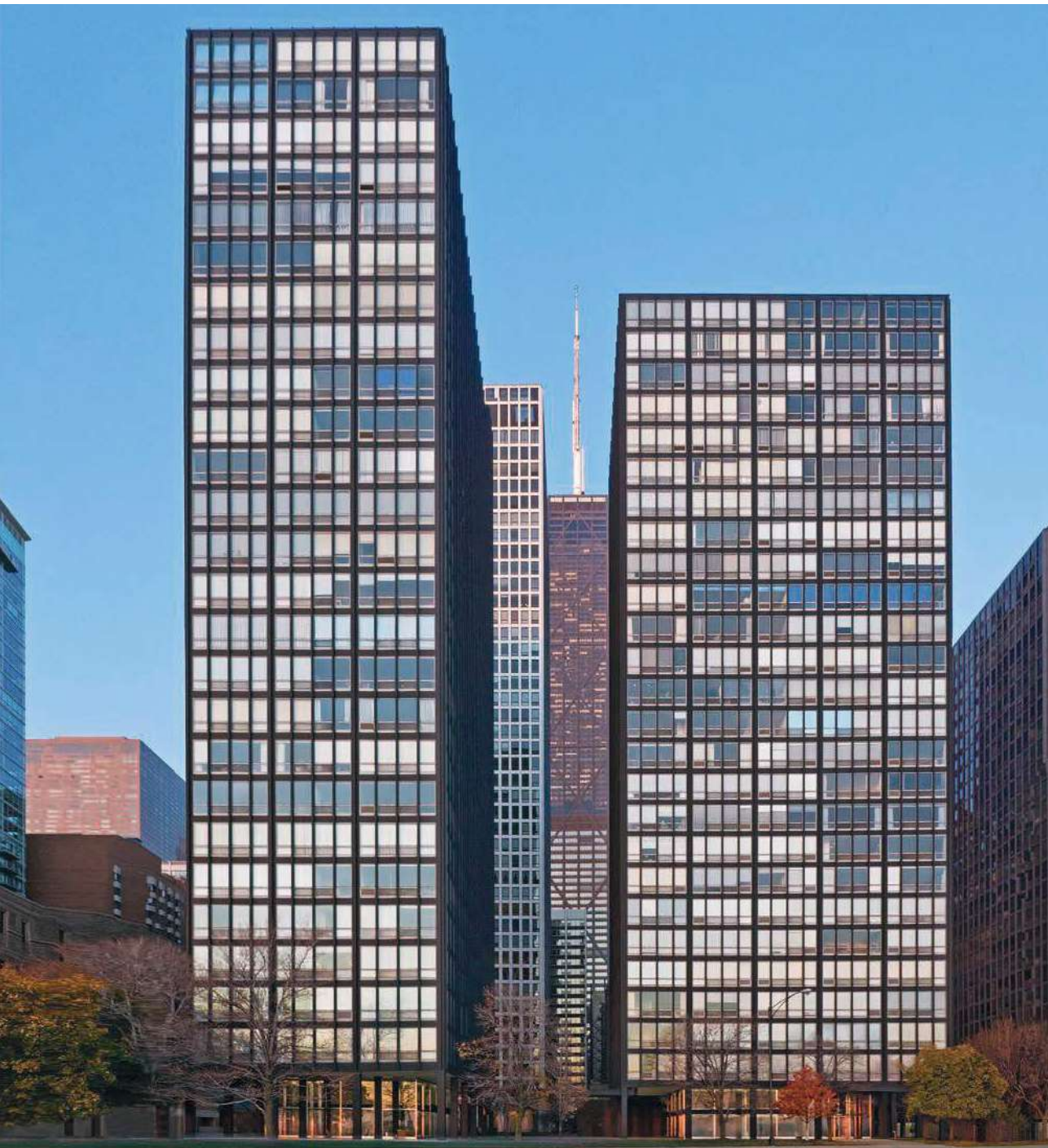
12 13 Ludwig Mies van der Rohe, Lake Shore Drive Apartments, Chicago, 1949-1951.
