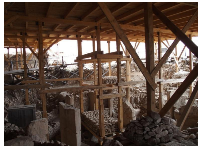
Figure 5. The wooden roof for protecting the artifacts.
