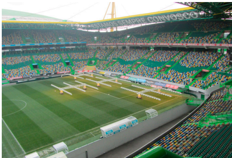
Figure 1. General view of the South grandstand.
