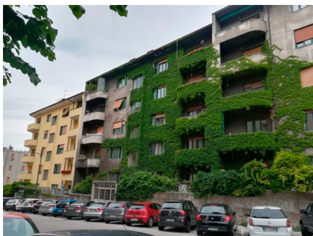
Figure 17. The facade of a house in Trieste City center. The climbing ivy was recently cut.
