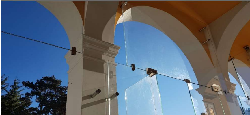
Figure 7. Glass partition assembly, detail view of the final construction (photo by A. Danelutti).
