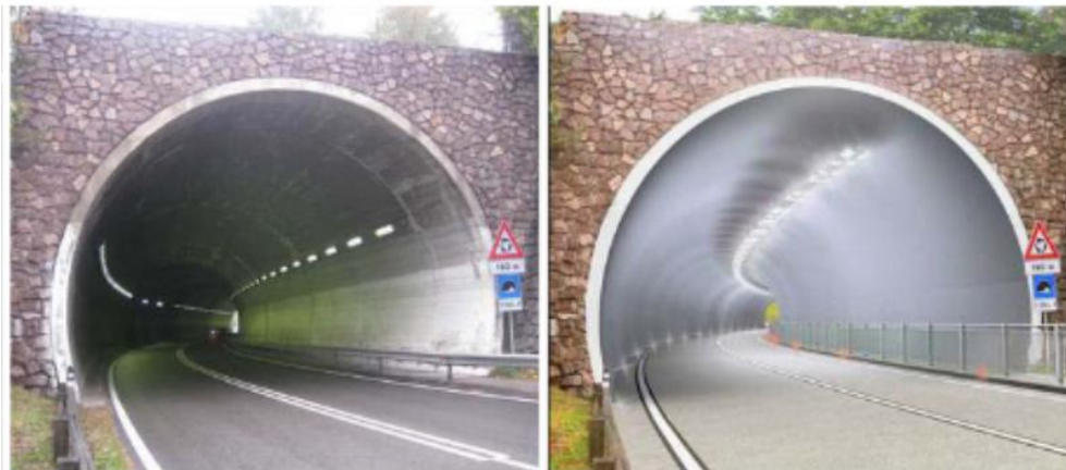
Figure 7.11. Black asphalt concrete (left) vs. clear mixture (right) paved in the tunnel [6.1].
