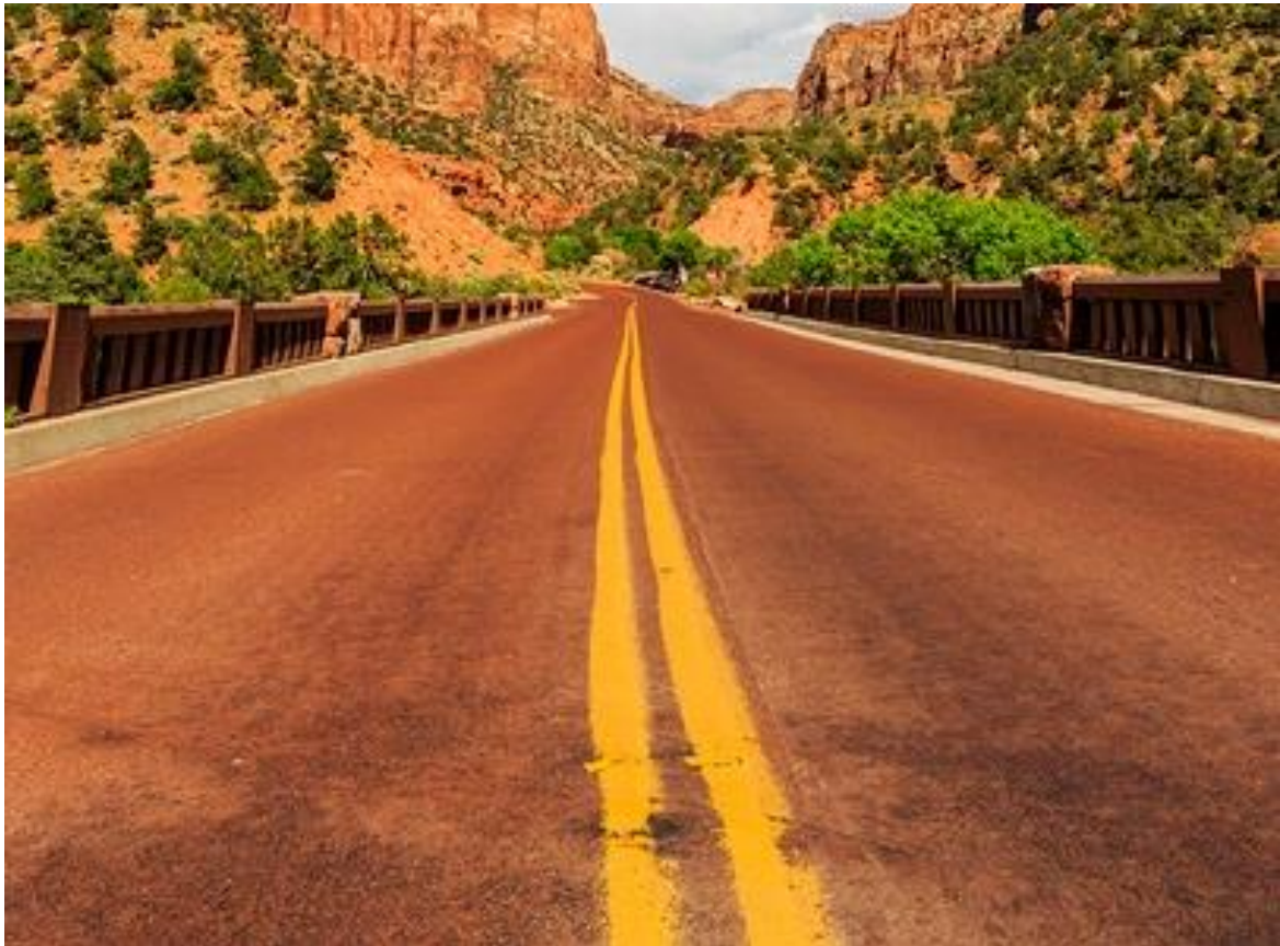
Figure 7.2. Colored asphalt pavement in a naturalistic context in Texas.
