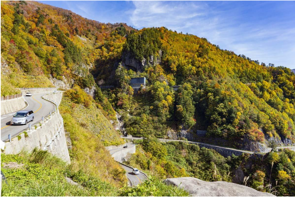
Figure 7.4. Clear road pavements located in Japan.
