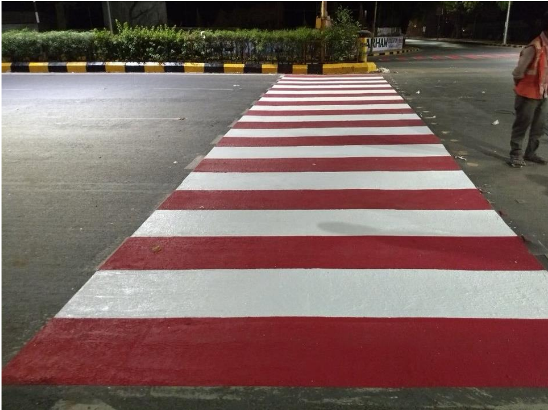
Figure 7.8. Example of red-painted pedestrian crossing.
