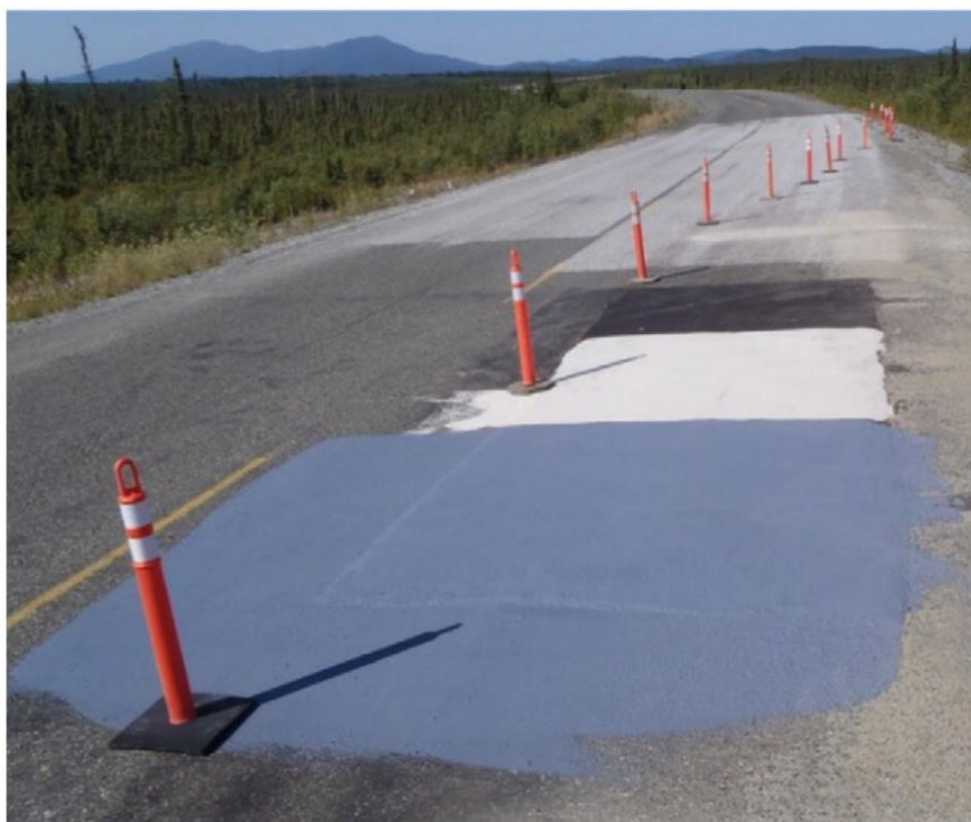
Figure 3.8. Real-scale application of flexible pavements for winter climate [3.17].
