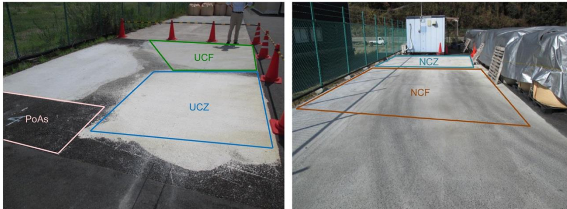
Figure 3.9. Trial sections for the analysis of pavement thermal responses [1.18].
