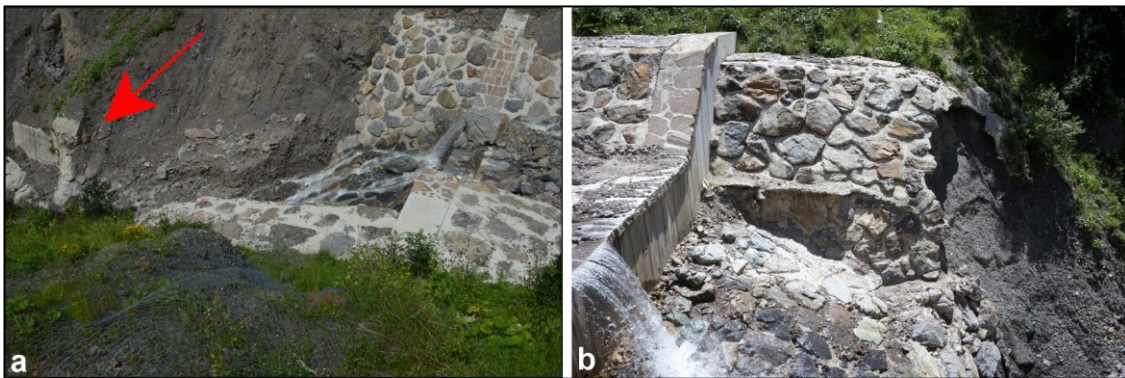
Figure 4.25: The erosion processes observed downstream of the lower check dams (n. 29). a) The erosion in 2016 after the debris-flow events. Another check dam (n. 28; Fig. 4.3d ) located 30 m further downstream, destroyed by debris flows in the recent past, is also visible (red arrow). b) Local scouring and erosion observed in June 2018 that undermined the stability of the hydraulic control works.
