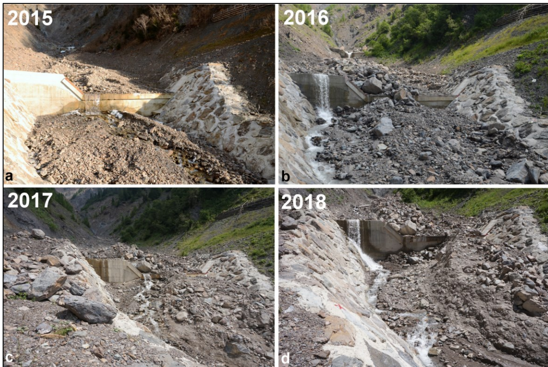
Figure 4.24: Sediment deposits at the site of the upper check dam (n. 30). a) 15 December 2015. b) 22 July 2016. c) 20 July 2017. d) 19 July 2018.
