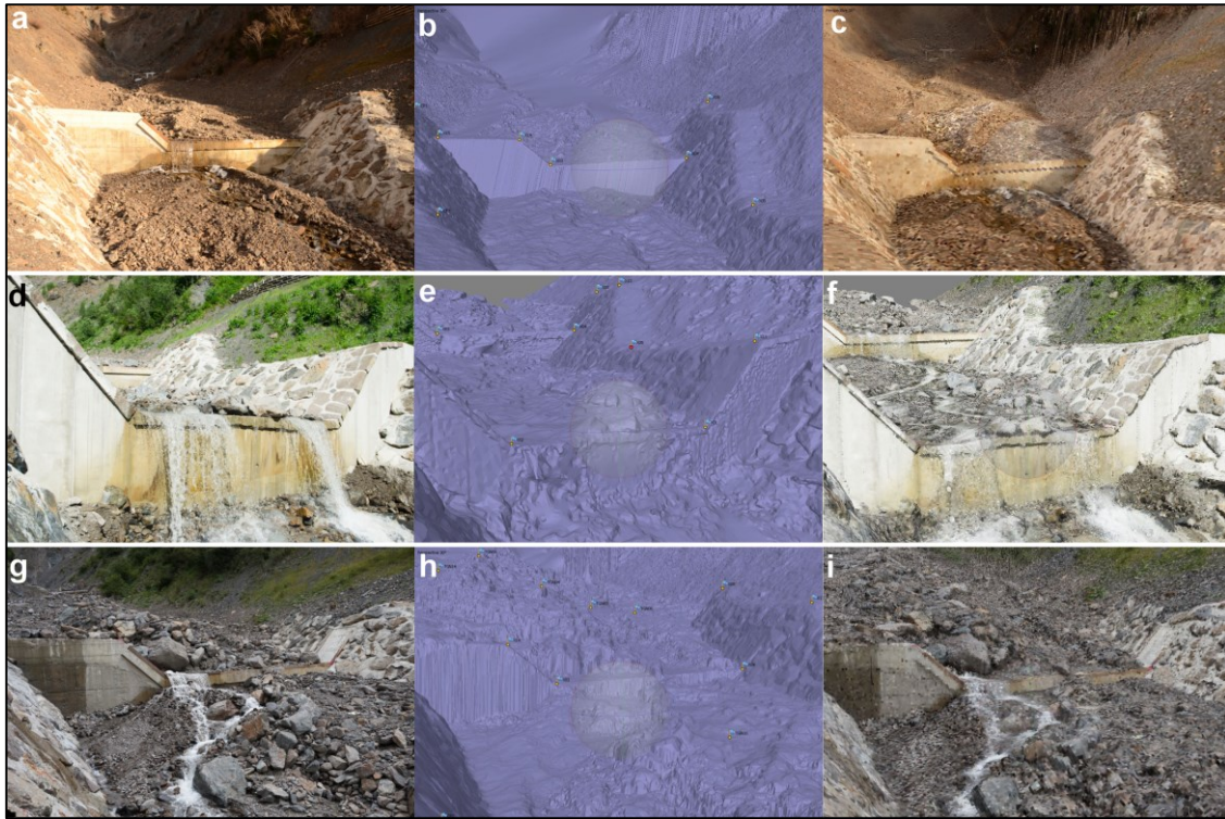
Figure 4.11: Example of comparison between the photos (used as input in SfM software) and 3D models (terrain and tiled model) obtained by Photoscan software for the SfM study area. a) The photo of the check dam (n. 30). Cucchiaro, December 2015. b) The terrain model that reconstruct 3D view of Figure 4.11a . c) The tiled model that reconstruct 3D view of Figure 4.11a . d) The photo of check dam (n. 29). Cucchiaro, June 2016. e) The terrain model that reconstruct 3D view of Figure 4.11d . f) The tiled model that reconstruct 3D view of Figure 4.11d . g) The photo of check dam (n. 30). Cucchiaro, August 2016. h) The terrain model that reconstruct 3D view of Figure 4.11g . i) The tiled model that reconstruct 3D view of Figure 4.11g .
