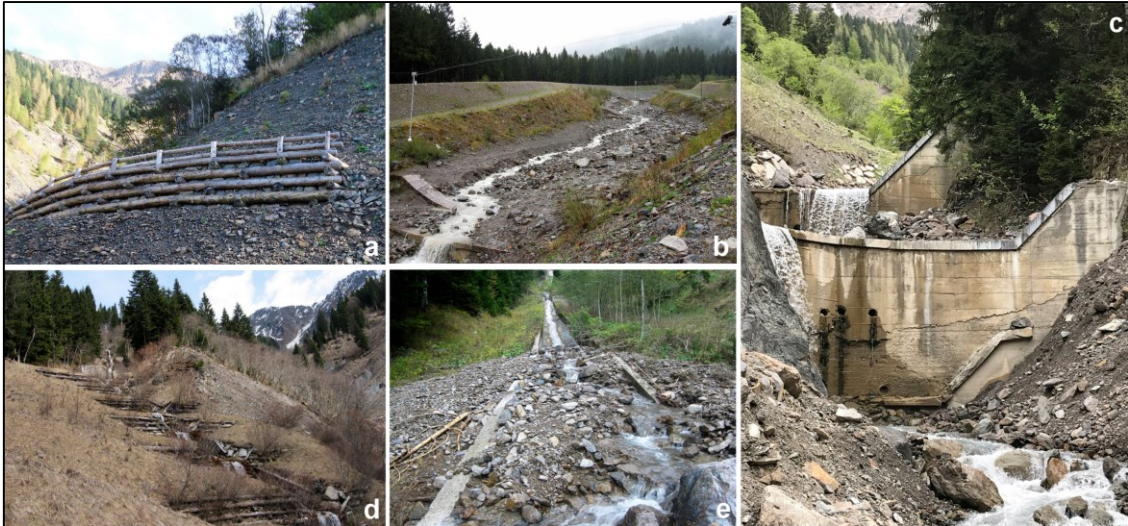
Figure 2.6: Torrent control works over time in the Moscardo catchment. a) Bioengineering interventions built in 2014 to stabilize a slope in the upper part of the Moscardo catchment. Cucchiaro 2014. b) Riverbanks stabilization in the lower part of the catchment close to the monitoring station in 2011. Blasone 2012. c) Example of reinforced check dams built in the 1980s along the main channel of the Moscardo torrent. Cucchiaro 2018. d) Sequence of wood and boulder check dams to stabilize the slope and channelize Rio Lares stream (Fig. 2.1). Blasone 2011. e) Canalization of Rio Lares stream after debris-flow events in 2012. The structure was built in the 1980s. Blasone 2012.
