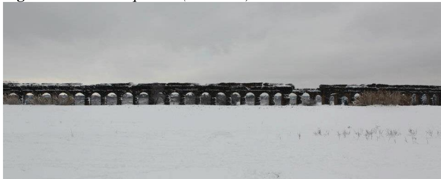
Figure 32. Roman Aqueduct (I sec. d.c.)
