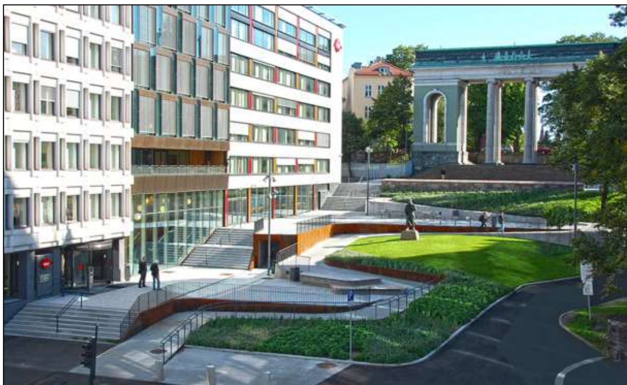
Figure 2. Schandorff Square view [6].
