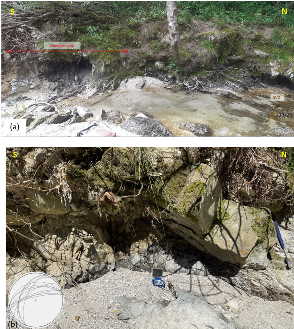
Fig. 4.9 – (a) Damage zone affecting the Eocene turbiditic unit (SVO) in the Torre riverbed (field stop n° 5, Figs. 4.1 and 4.7). In the stereographic plot the intense cleavage affecting marly SVO layers (b).
