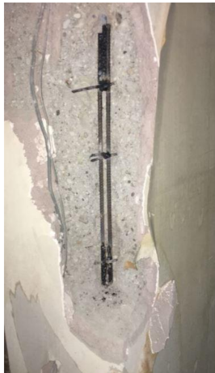
Fig. 20. Extraction of reinforcement bar.
