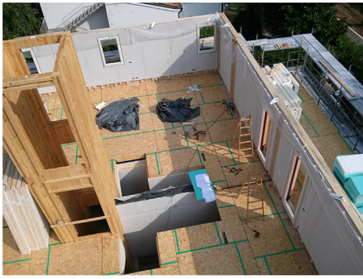
Fig. 11. Multi-storey glulam with top boards building.
