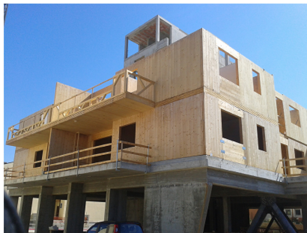
Fig. 1. Multi-storey Cross Laminated Timber building.
