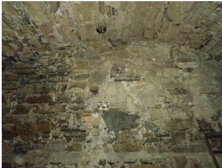
Figure 3-47: Stone masonry visible in the room A004 of the basement.
