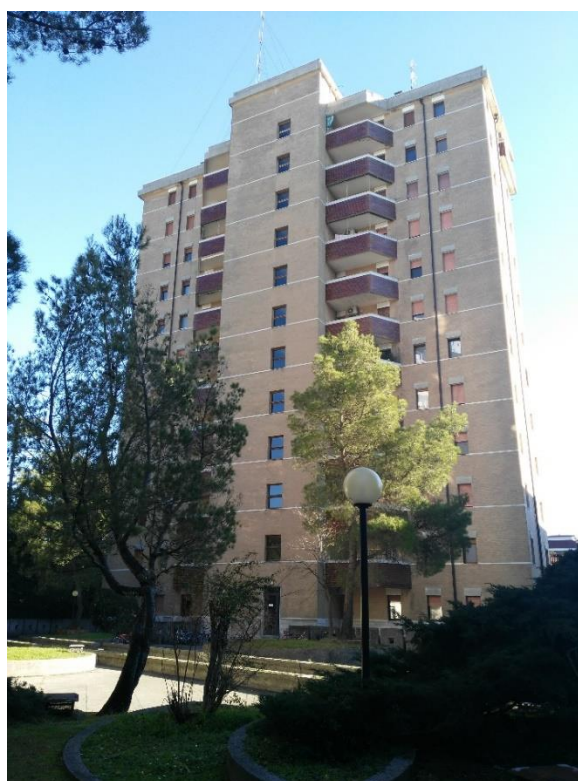
Figure 3-1: View of the back façade of case study RC building 1.
