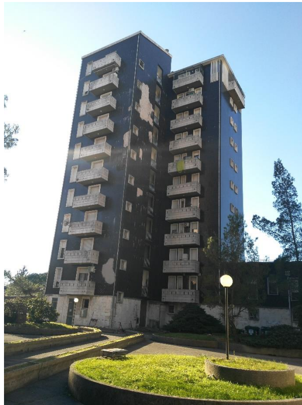
Figure 3-25: Side view of case study RC building 2.
