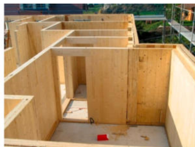
Fig. 4. Shear-wall structure example: CLT structures ( www.unikore.it ).
