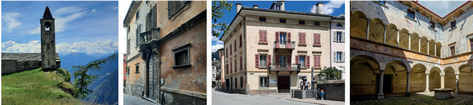
Fig. 1 Image of the case studies: San Romerio church, Tirano (Brusio, Switzerland); Visconti Venosta palace, Tirano, Italy; Semadeni palace, Poschiavo, Switzerland; Besta palace, Teglio, Italy (left to right).
