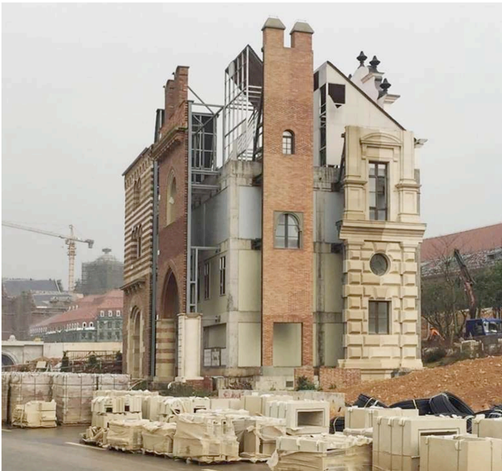
Facade test for Huawei's European themes campus in Dongguan, 2019: the architectural schism between cladding and structure as a metaphor between interpretation and reality?
