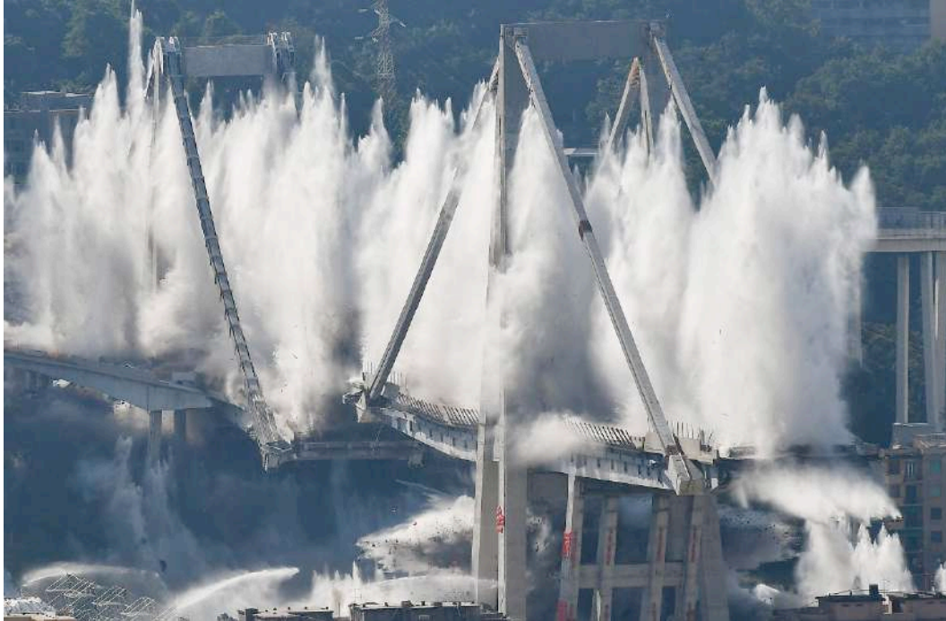
The demolition of Morandi bridge, Genoa, 2019.
