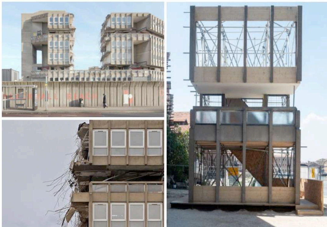
Top: demolitions of modernist housing developments.
