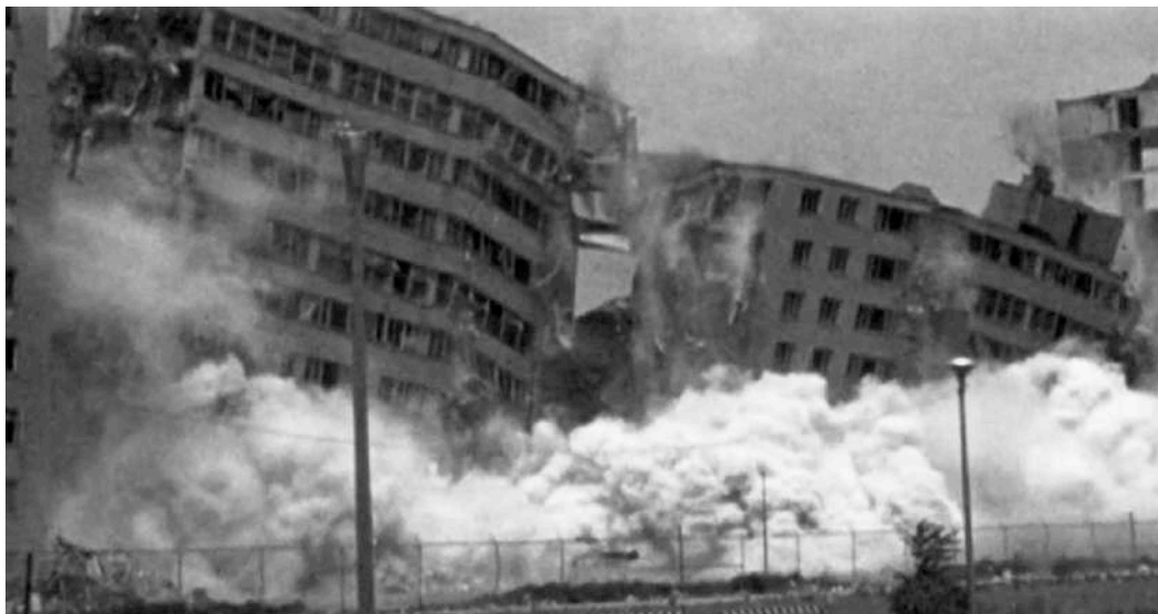
The first demolitions of Pruitt-Igoe complex, 1972.
