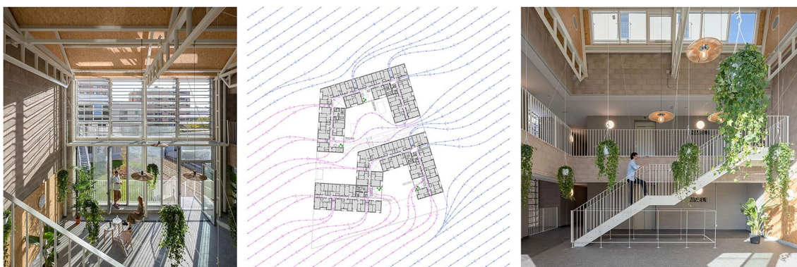
Fig. 3 TAA's social housing in Carabanchel views of a so-called "social condenser" and general floor plan showing the building's relation to cool nocturnal winds (© Javier y Alia García-Germán and ©TAA's totem arquitectos asociados)
