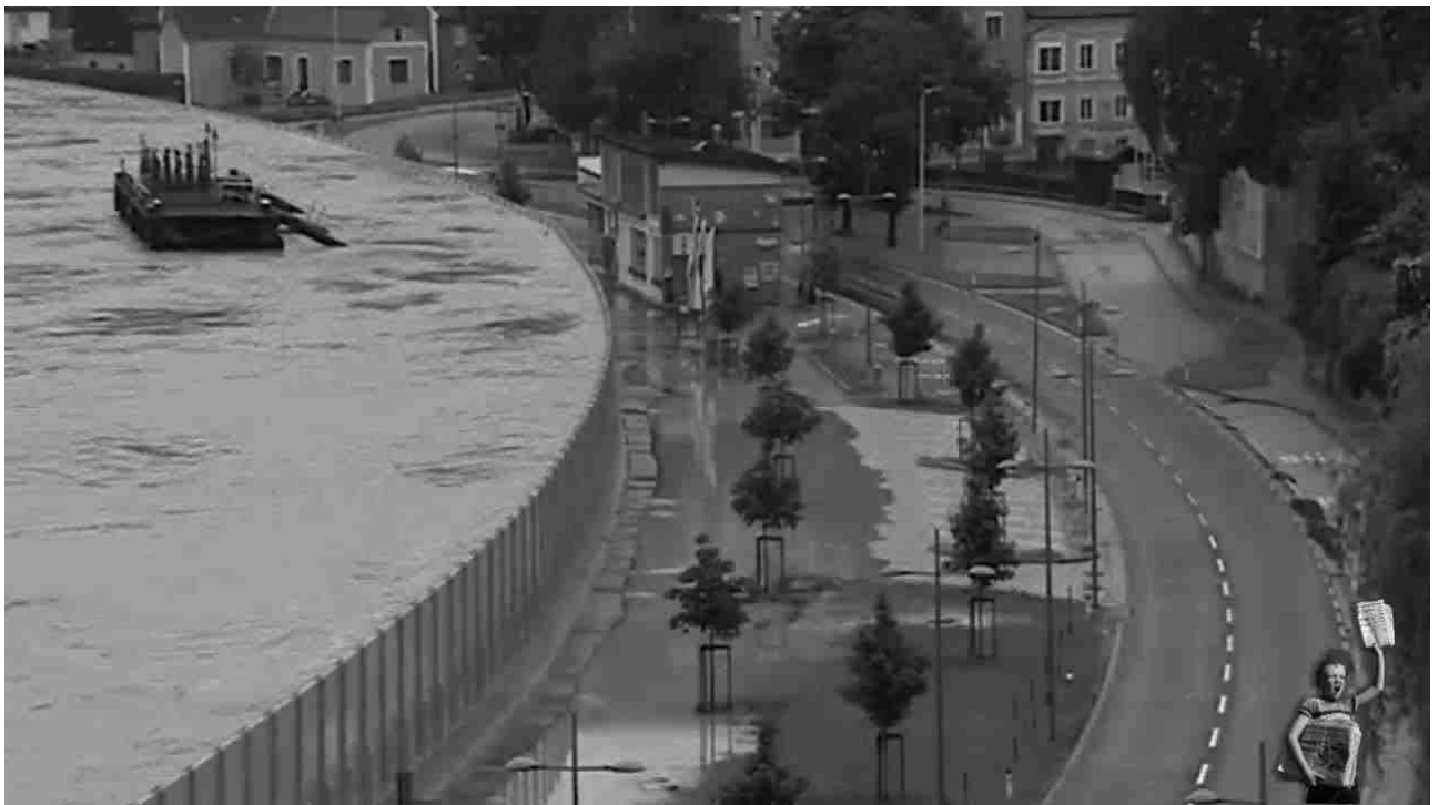
Figure 3: Mobile flooding protection structures such as those in Grein (Wachau) on the Austrian Danube can increase flood peaks and inundation risk downstream (source: Robert Zinterhof)
