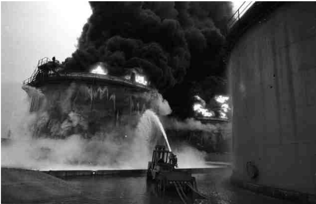
Figure 12: Bombardment of Novi Sad 1999 destroyed infrastructure and oil tanks leading to long-lasting environmental hazards (source: Darko Dozet).
